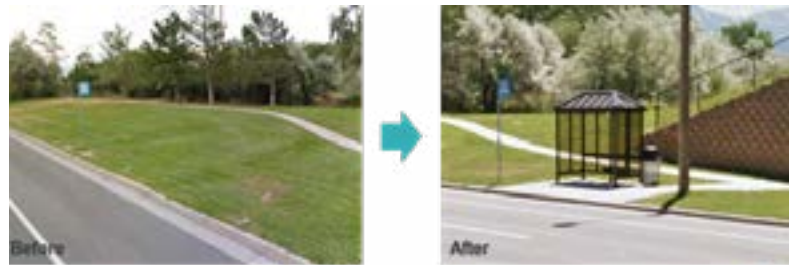
Image 51. Bus Stop Access (Source: TriMet) (top)
