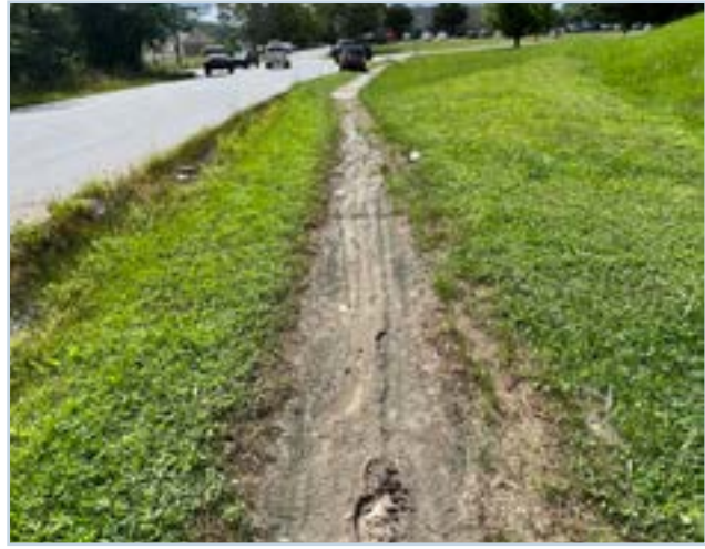
The existing sidewalk between Lakewood Road and Sam's Club is overgrown and full of sediment, indicating a drainage issue.
