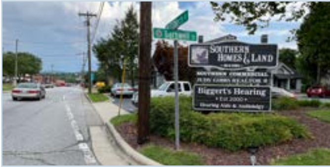
Utilities will require additional sidewalk width or utility strip to ensure that pedestrians have a minimum of 4 feet to pass around obstacles.
