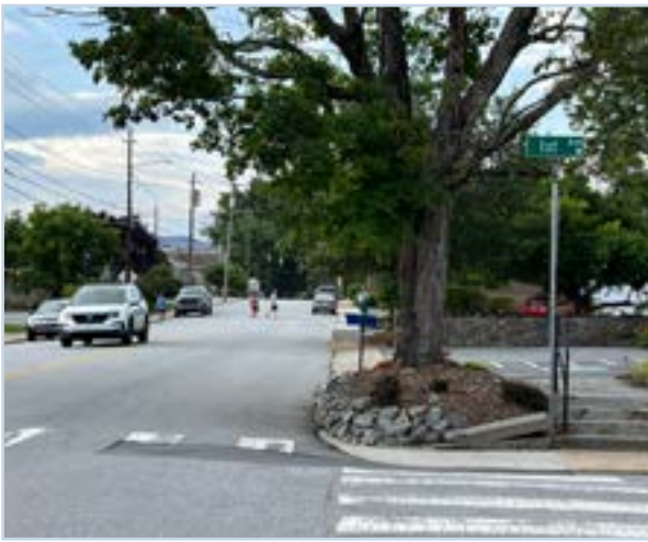
This missing connection north of 1st Avenue makes it hard for someone in a wheelchair or pushing a stroller to turn the corner. See also people in the background crossing midblock to access 2nd Avenue West.
