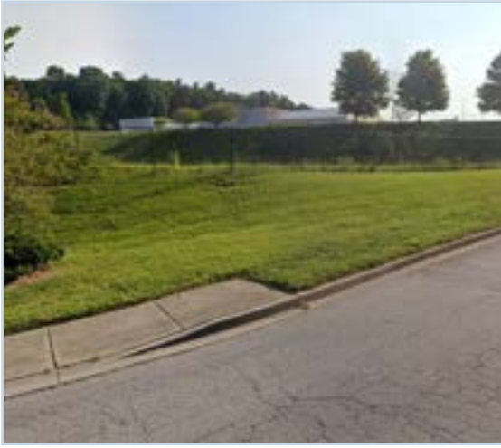
The sidewalk from Lakewood Road ends before reaching Walmart, limiting accessibility and forcing people to choose between walking in the grass, on the roadway, or not at all.
