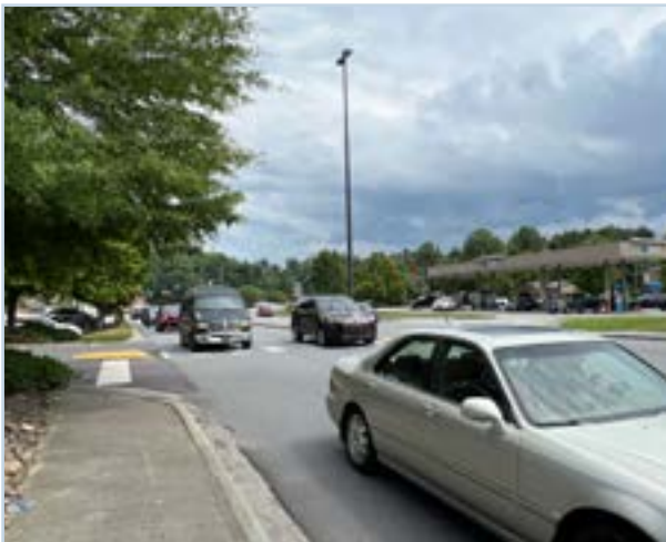
The existing crossing near Chick-Fil-A and US 64 driveway has high traffic volumes and is wide. This crossing should be relocated and updated to include ADA ramps and safety countermeasures.
